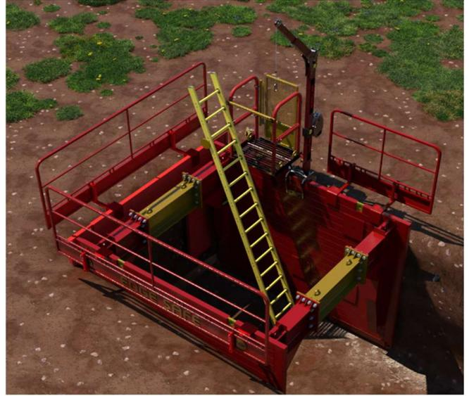
10. Safety equipment should now be installed on the box, if Endsafe panels are to be used then these should be lowered into position, prior to placing back fill behind them. Once a safe means of access is installed and subject to a final inspection the excavation is now safe to enter.
