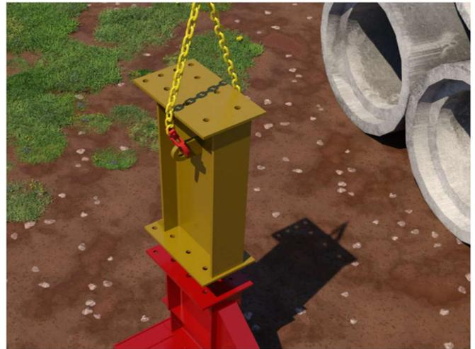
4. Connecting bolts can now be installed, ensure all nuts and bolts (10No. M24x70 each end) are securely fastened prior to removing the handling chains. Repeat this process for the remaining strut components. To avoid the need to work at height if multiple strut extensions are required then these should be connected prior to being installed onto the box.
