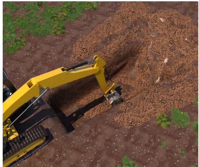
8. The trench should be dug to full depth to the required dimensions, allowing for a safe batter at either ends of the box. The ground must be self-supporting in the short term to allow the box to be installed. It is recommended to slightly overdig the trench to ease with lowering the box in.
